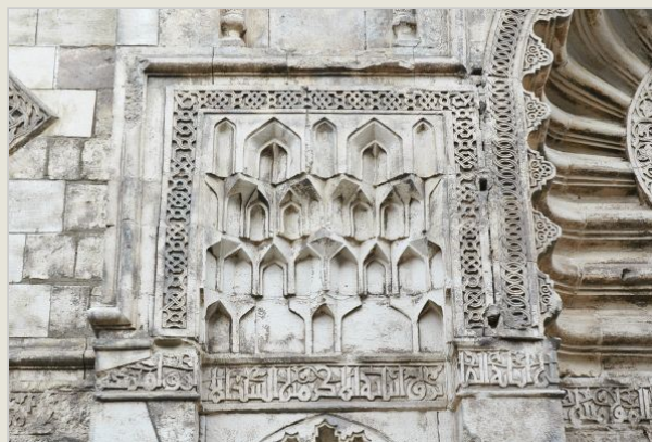
Figure 5.8 Restored muqarnas panel from the façade of the Aqmar Mosque, 1125. Cairo.
